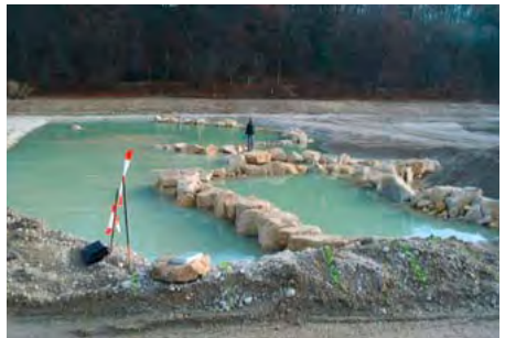
Ground ramp under construction: the staggered structure consisting of bars and pools is clearly recognisable. The base consisting of stones measuring 40 to 60 centimetres under the large stone blocks is also clearly visible.
