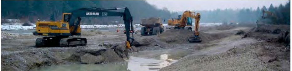
Hidden bank revetment: prefabricated river bank with filled gravel banks
