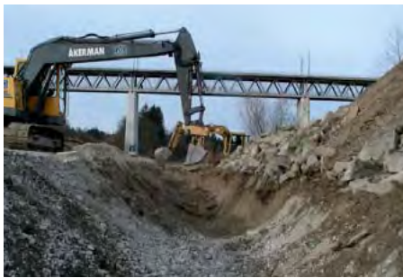
Dynamically developing bank with reverse defence system (in this case in the form of a trapeze-shaped security ditch)
